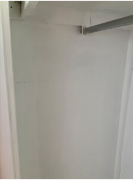
Horizontal crack at wardrobe. Pre-existing condition.
