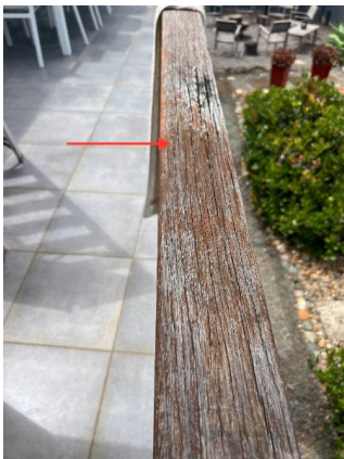
Timber handrail is deteriorating
