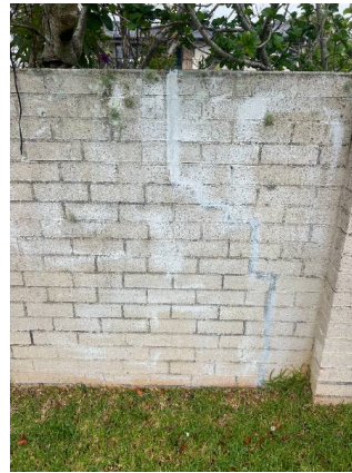
Minor cracks in brick fence have been patched.
