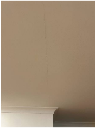
Cracks in ceiling
