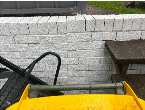
Cracks in brick retaining wall have been patched.
