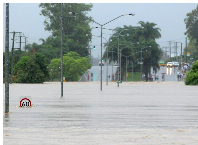
Caboolture River at Morayfield Road January 2011
