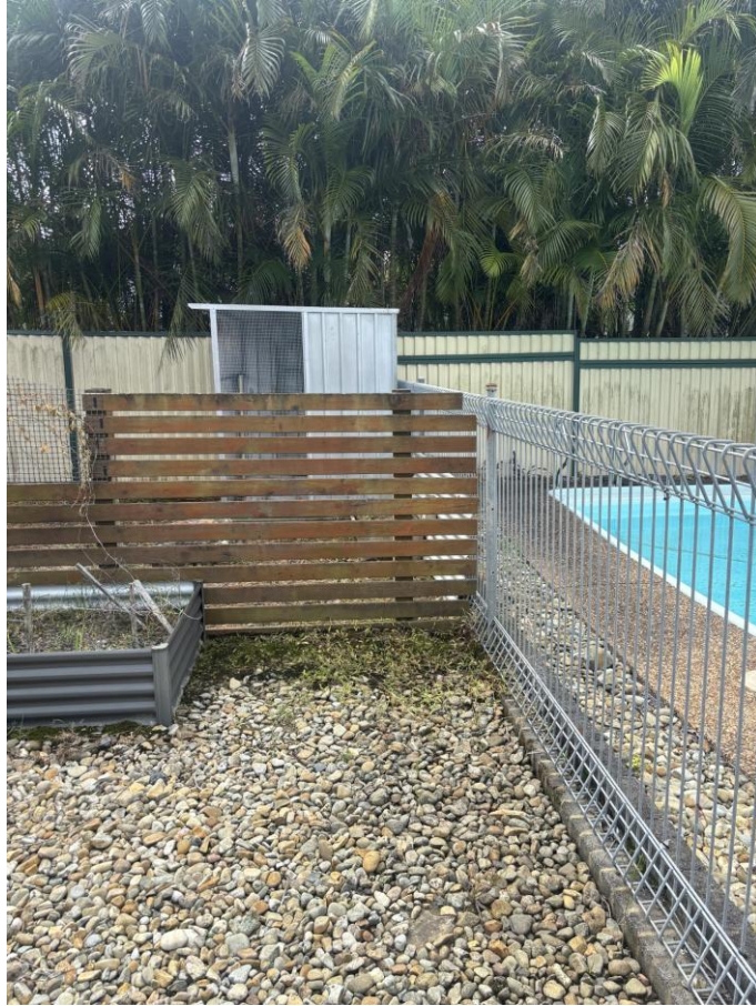
Image 2: Screen with gaps bigger than 10mm in no climb zone. Remove/cut back screen 900mm away from pool fence
