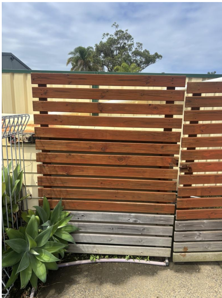
Image 1: Screen and gate needs to be removed as it has gaps greater than 10mm and can be used to climb on to pool filter cover
