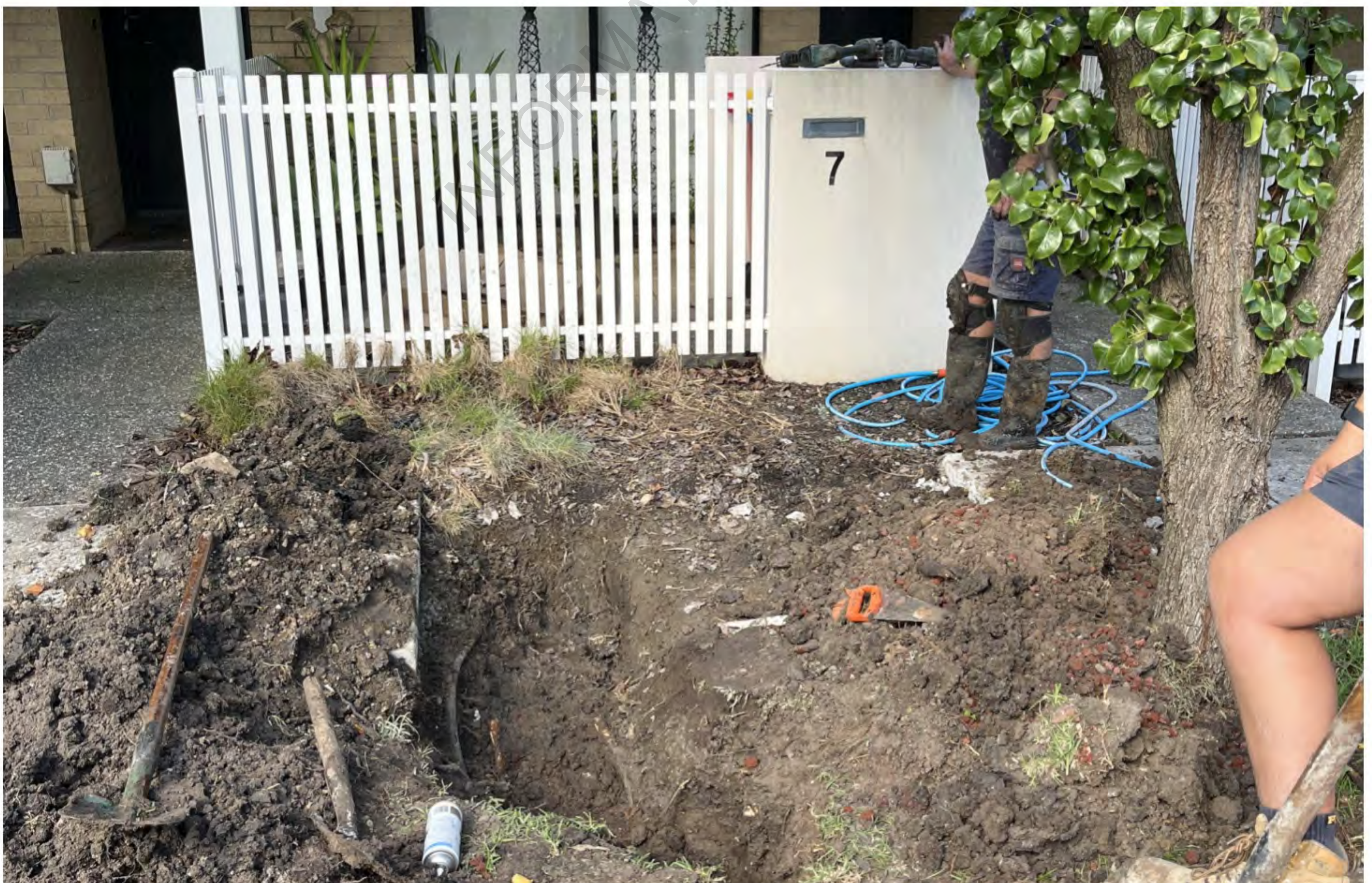
Photo 2: Excavation to find water connection
