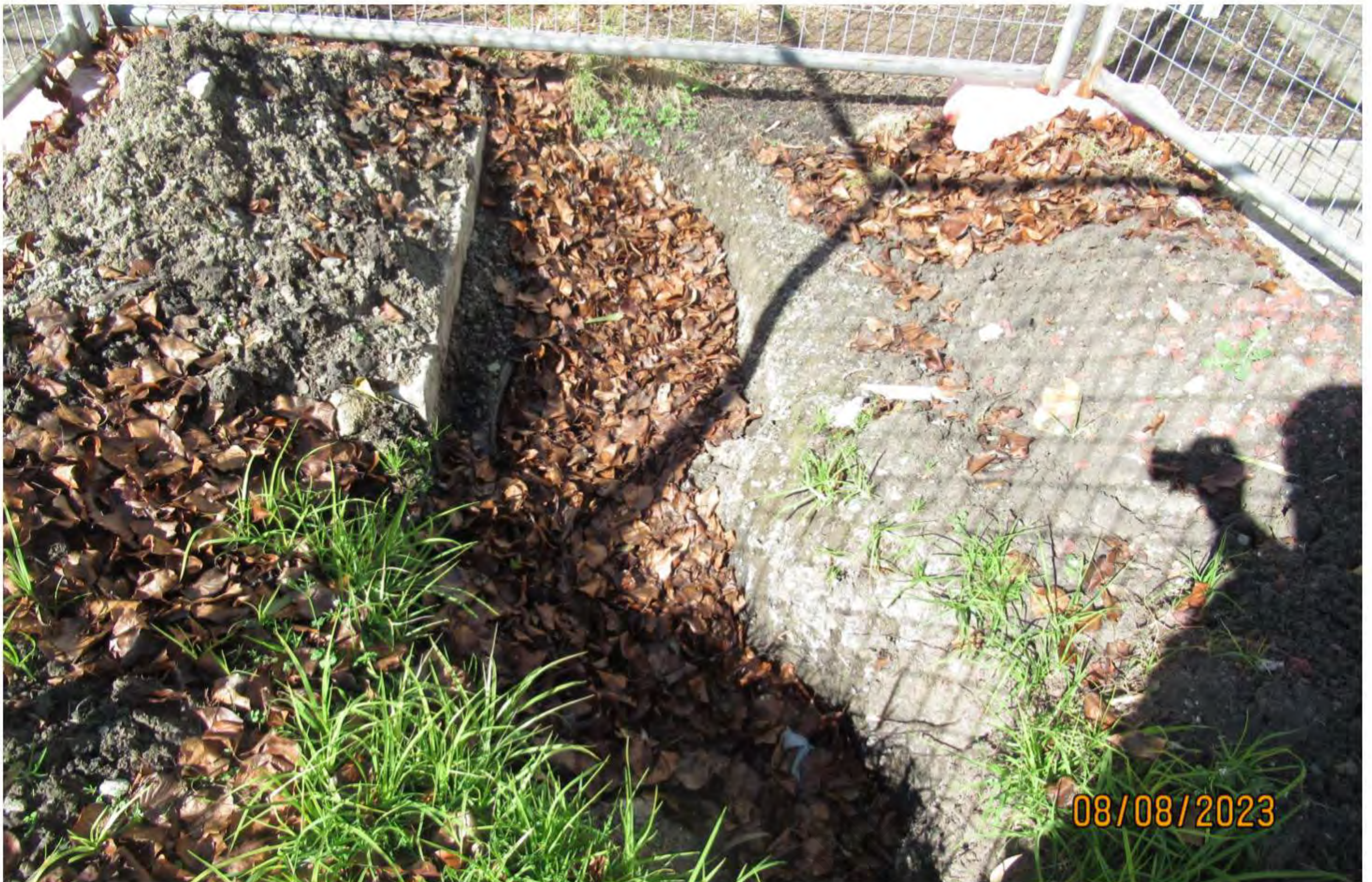
Photo 1.45: Excavation in front of 7 Gorman Drive
