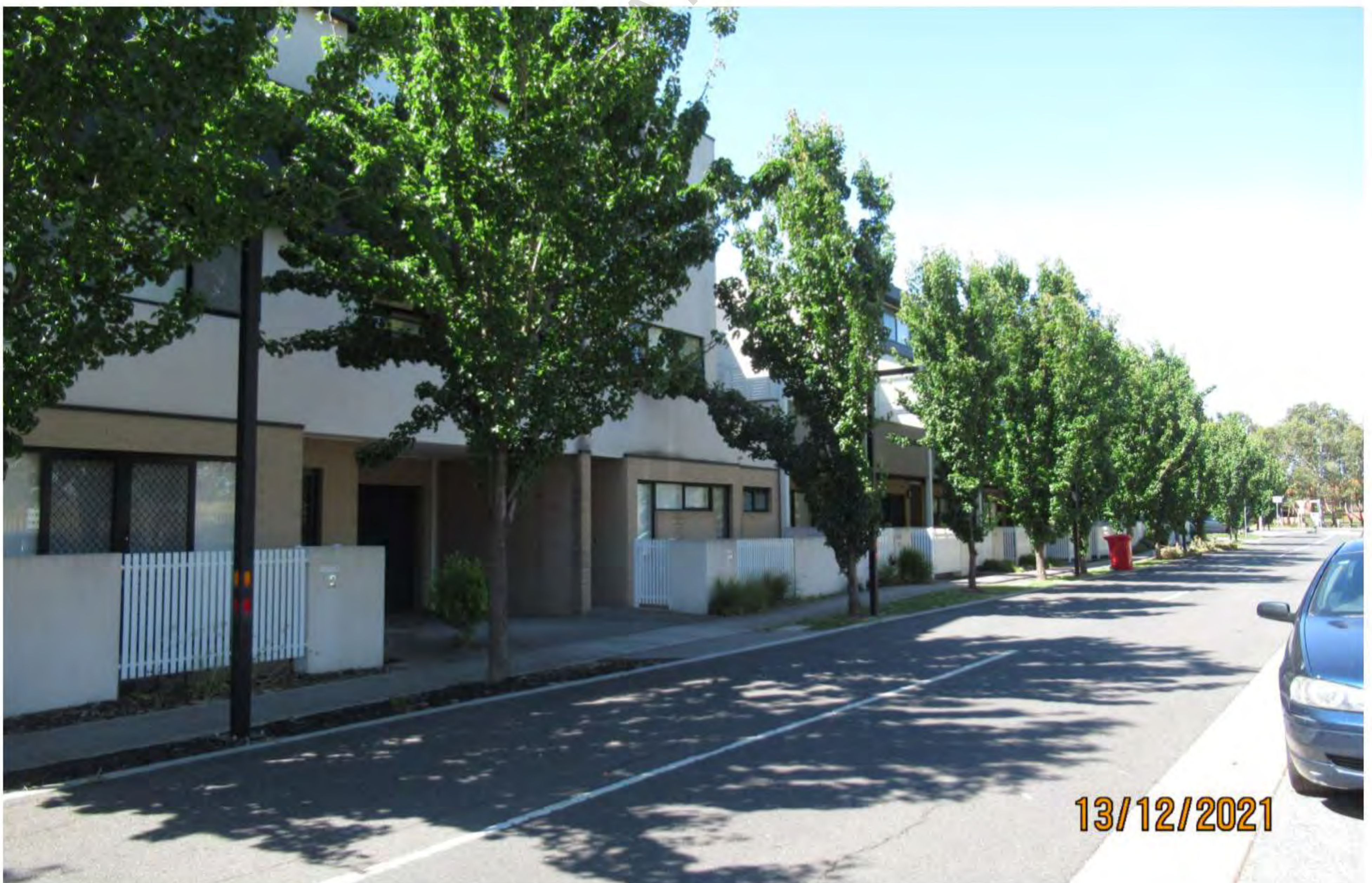
Photo 1.12: Longitudinal cracks in far side of Gorman Drive Leg A
