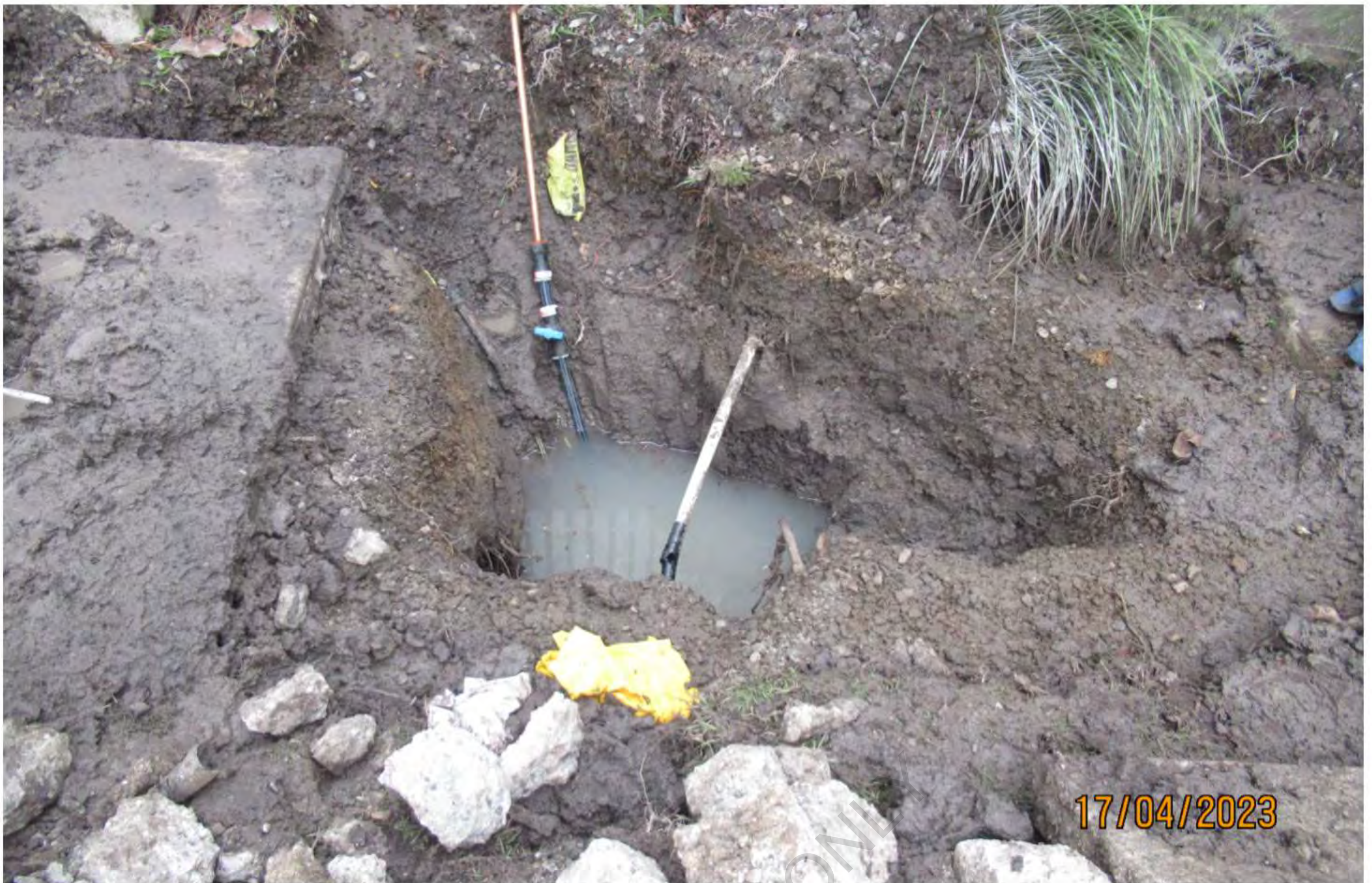
Photo 1.27: Repairs carried out to leaking water pipe
