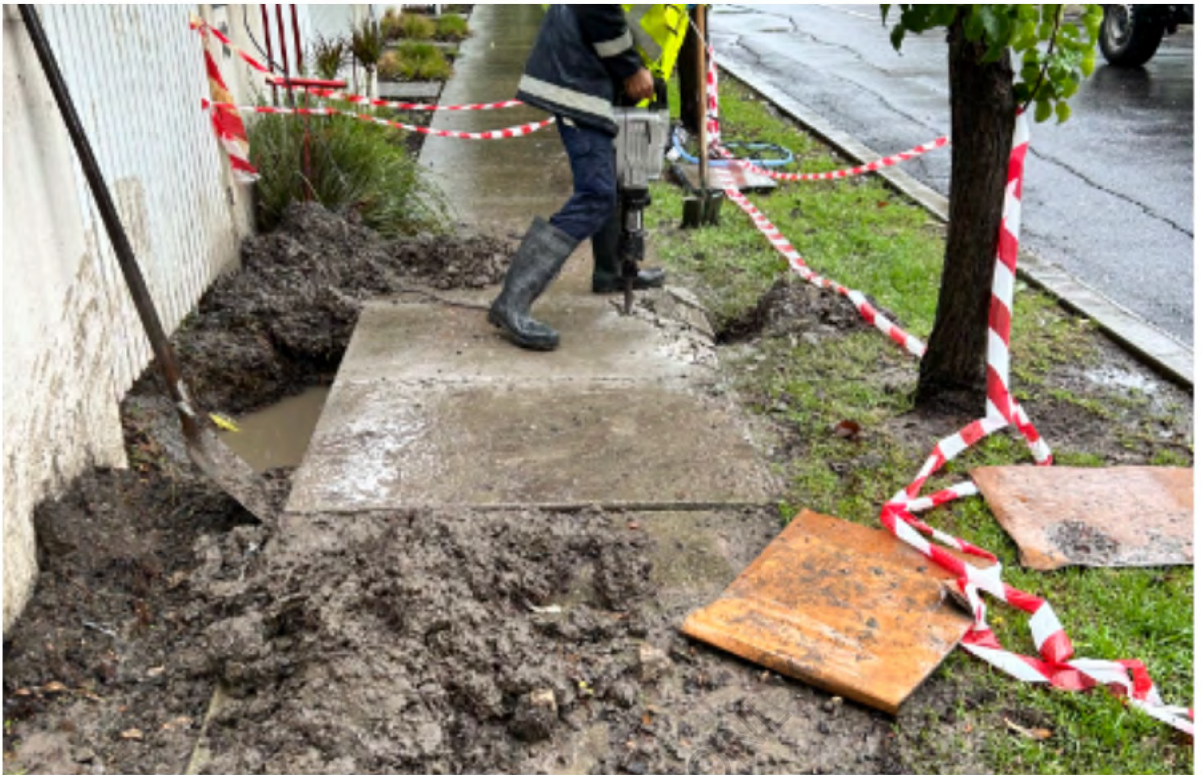
Photo 2.3: Excavation to find cause of leakage
