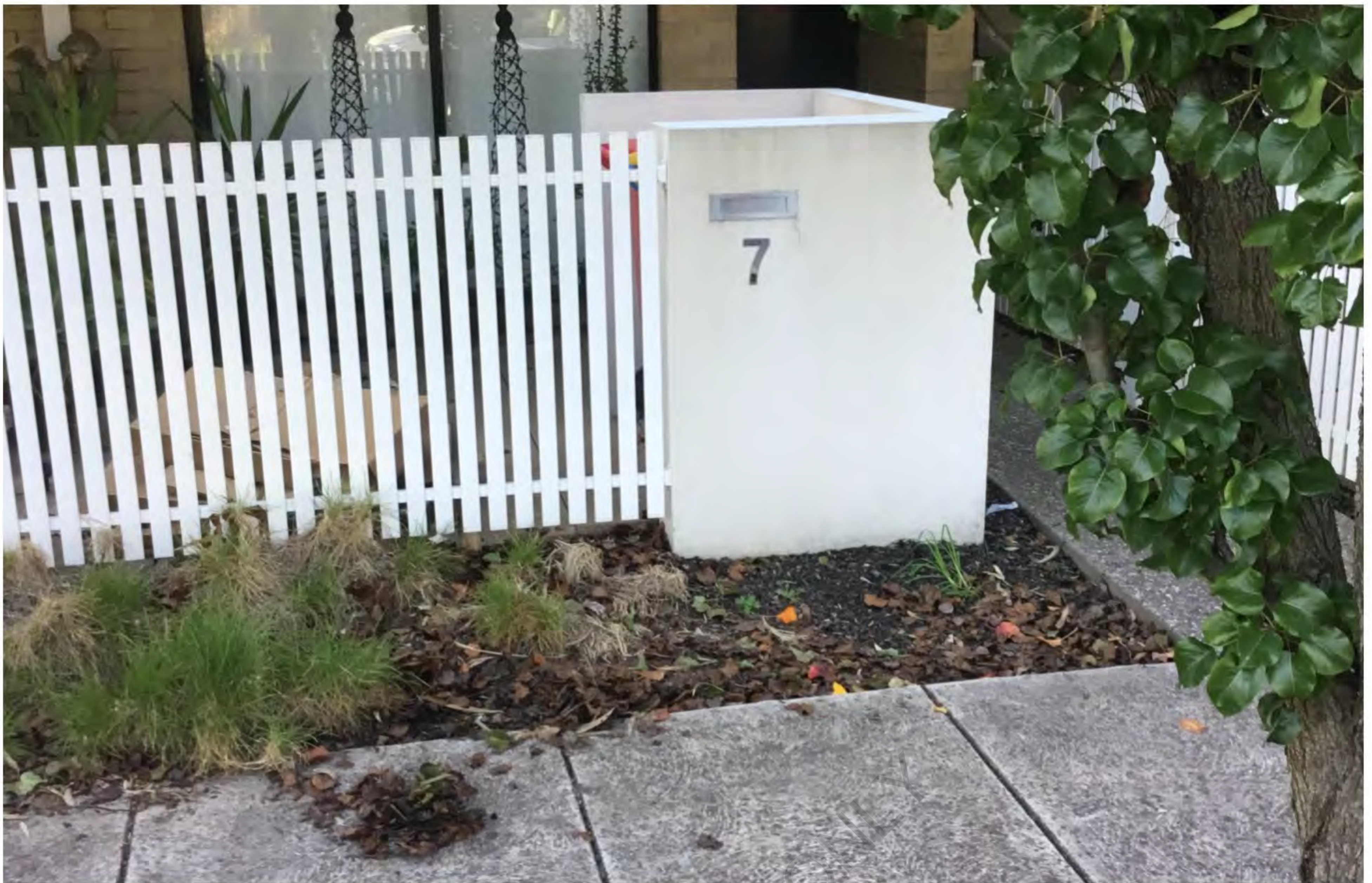
Photo 1: Investigation at 7 Gorman Drive
