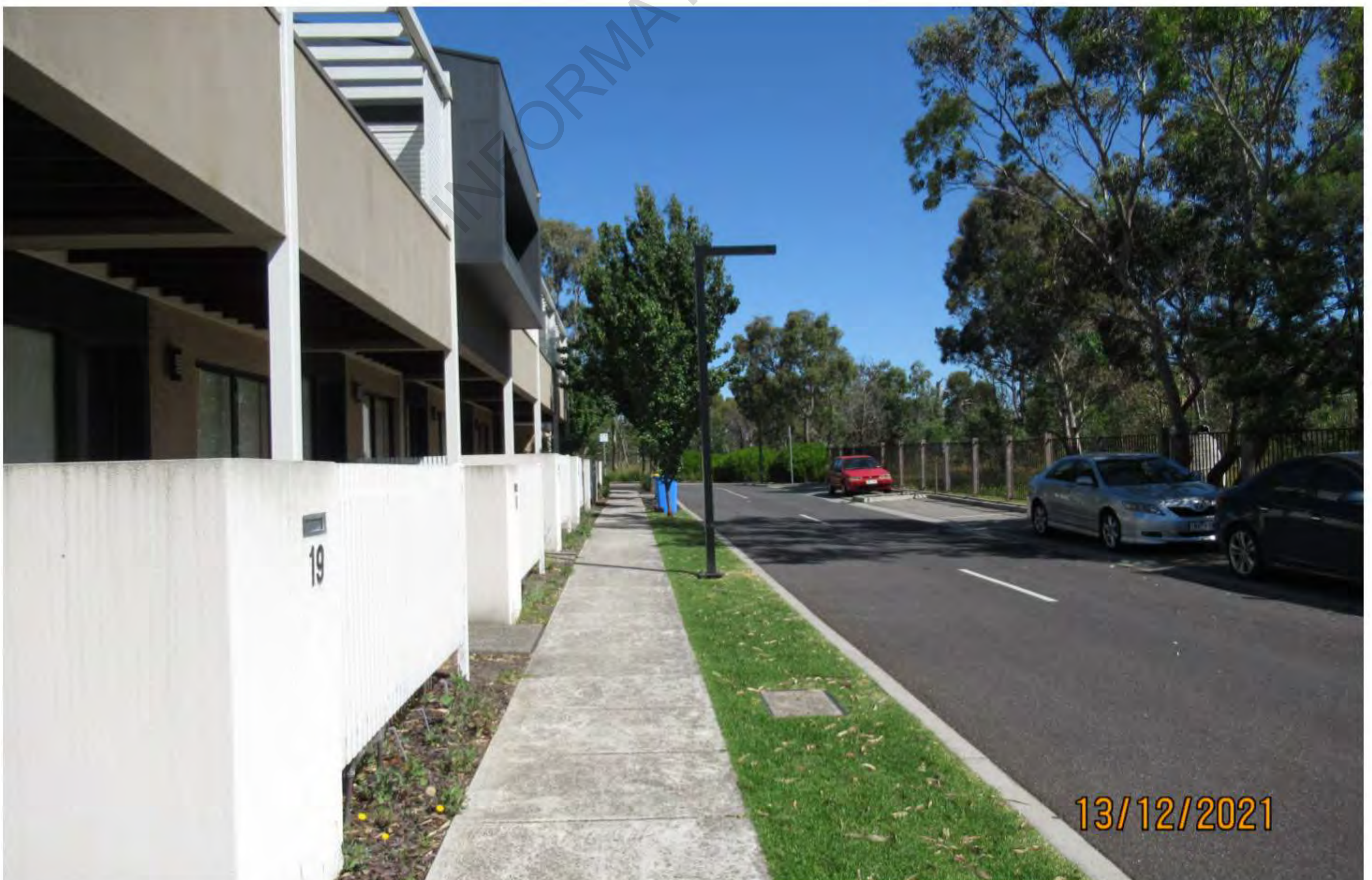
Photo 1.2: Gorman Drive looking north-west toward north corner
