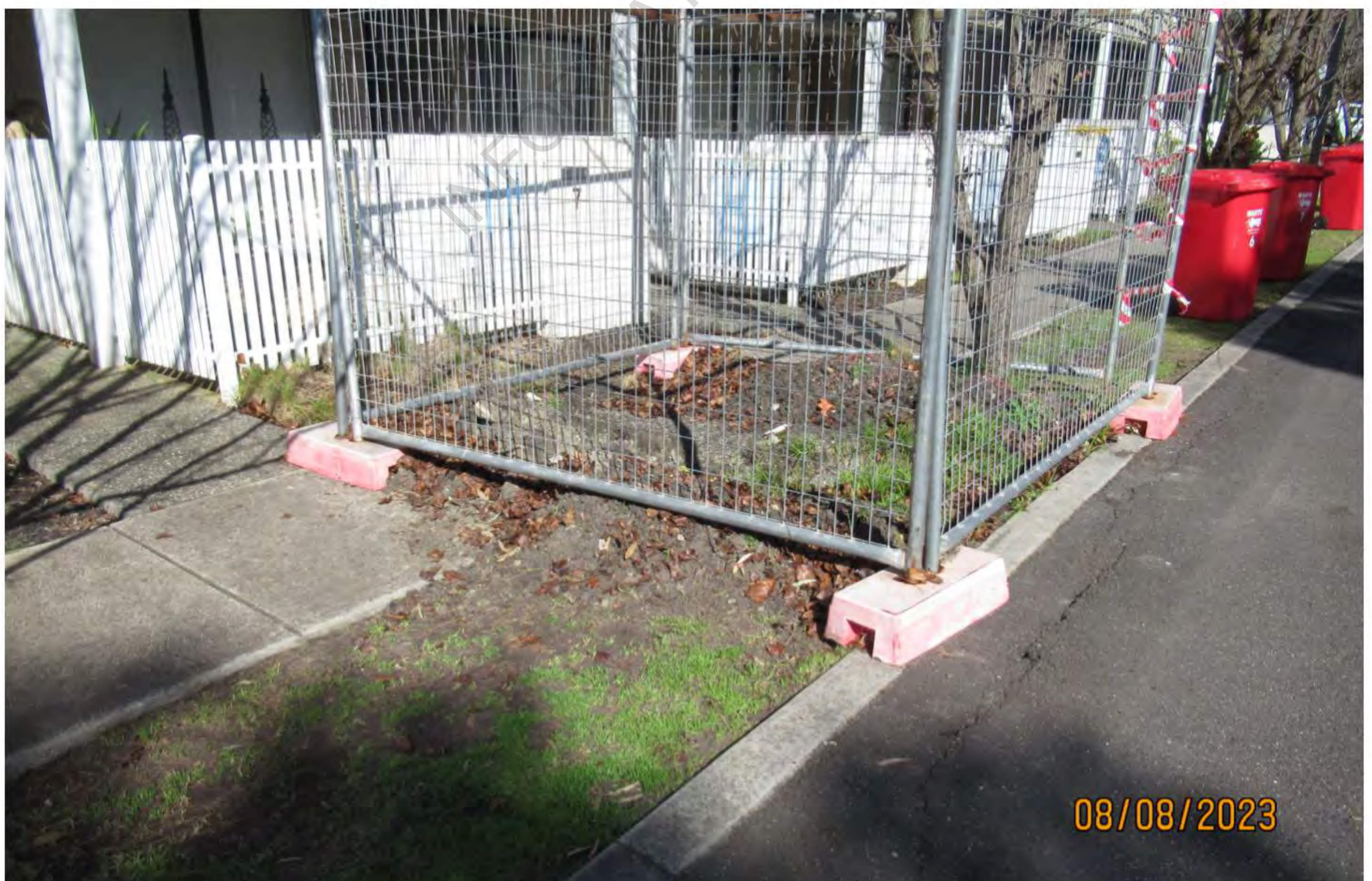
Photo 1.44: Location of excavation in front of 7 Gorman Drive
