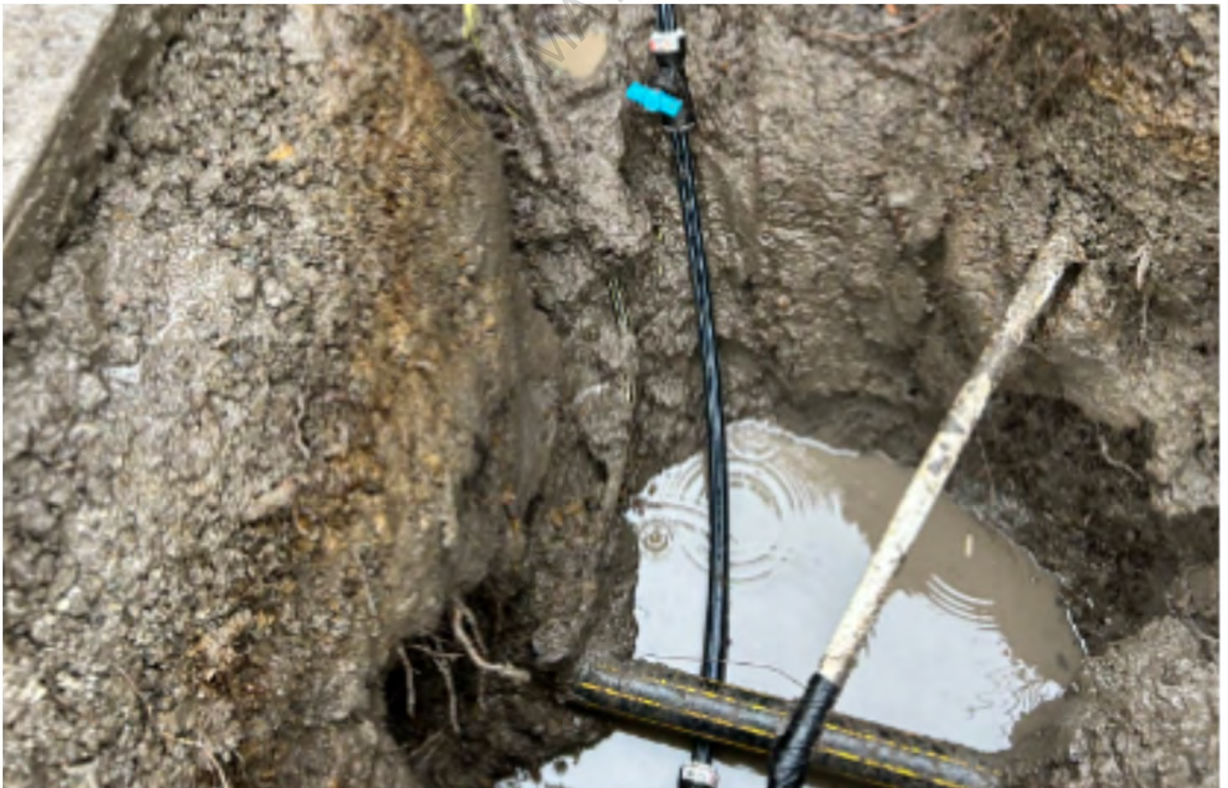
Photo 2.4: Excavation to find cause of leakage
