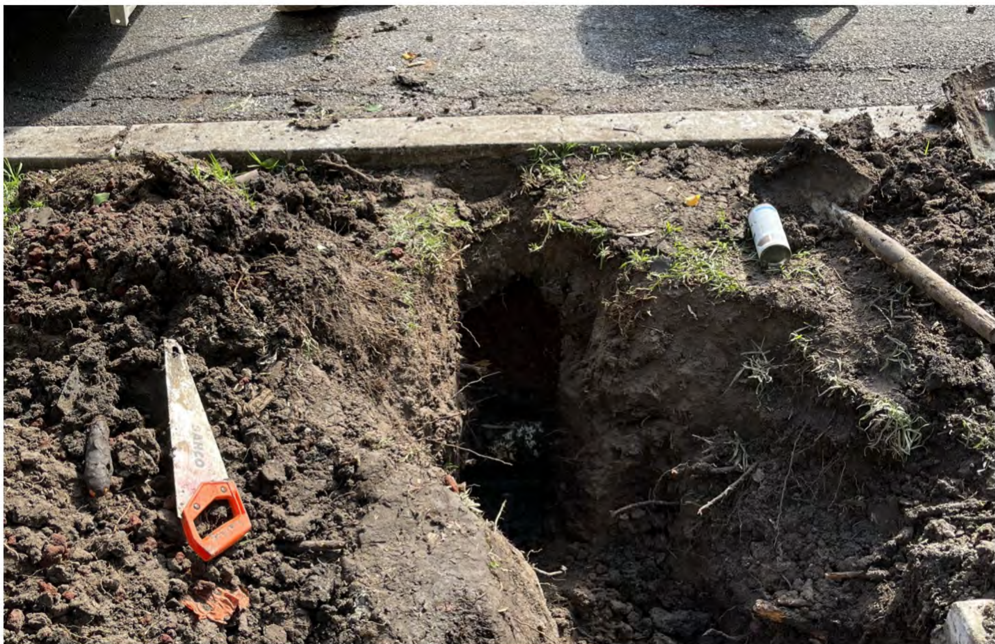
Photo 3: Excavation to find water connection
