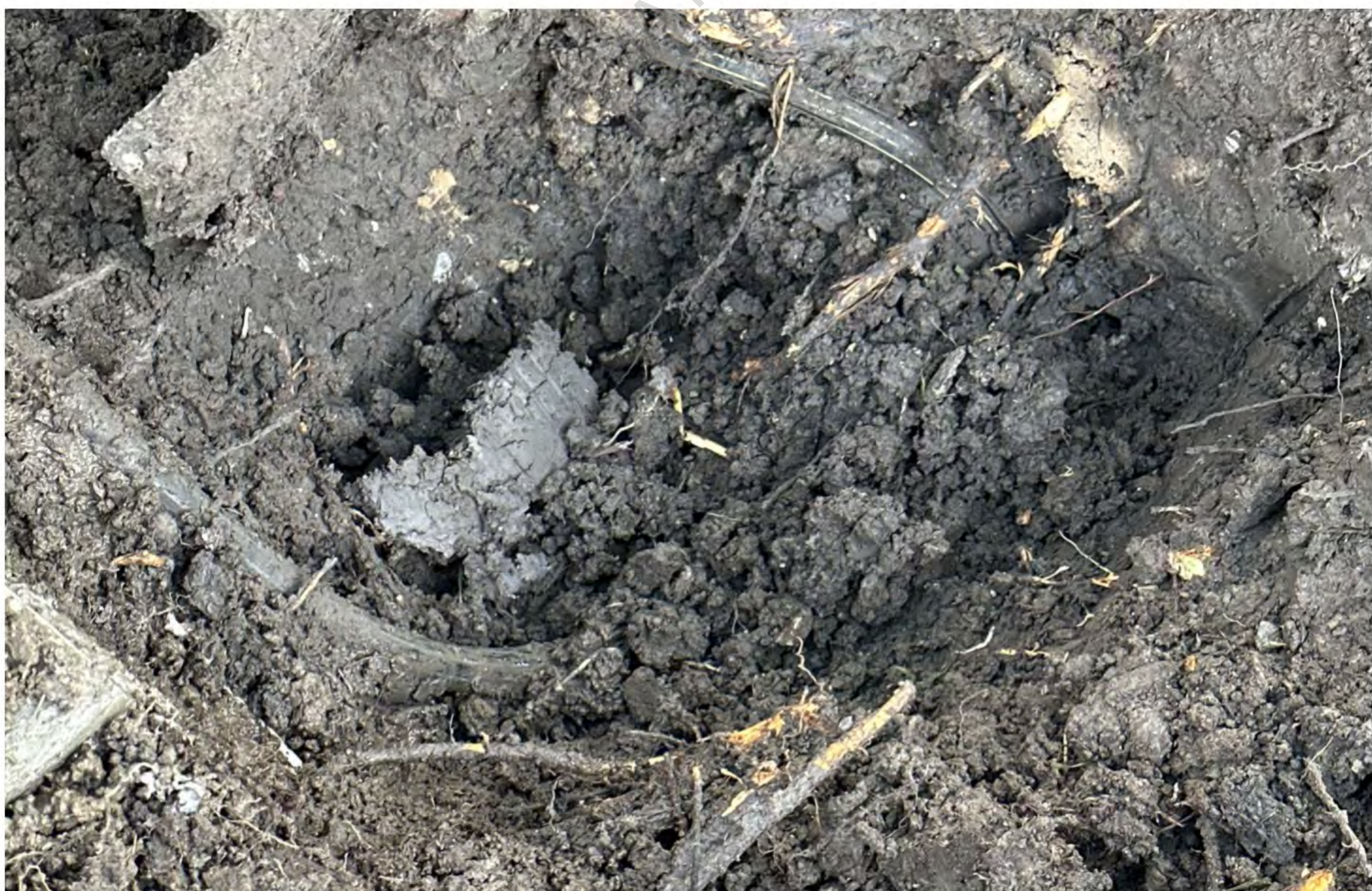
Photo 4: Excavation to find water connection
