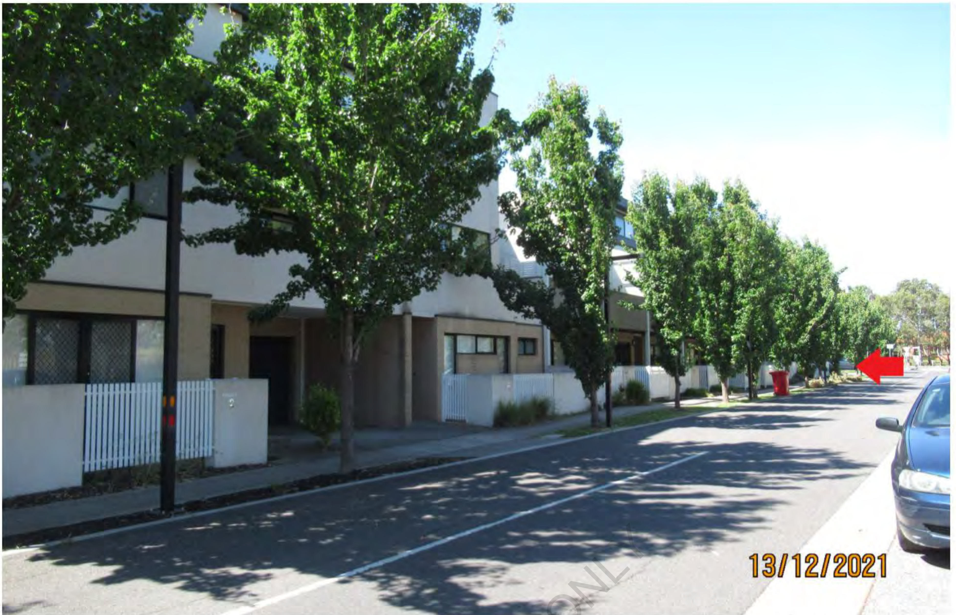
Photo 1.5: Gorman Drive looking south-west toward Bush Boulevard; red arrow indicates Olsen Walk
