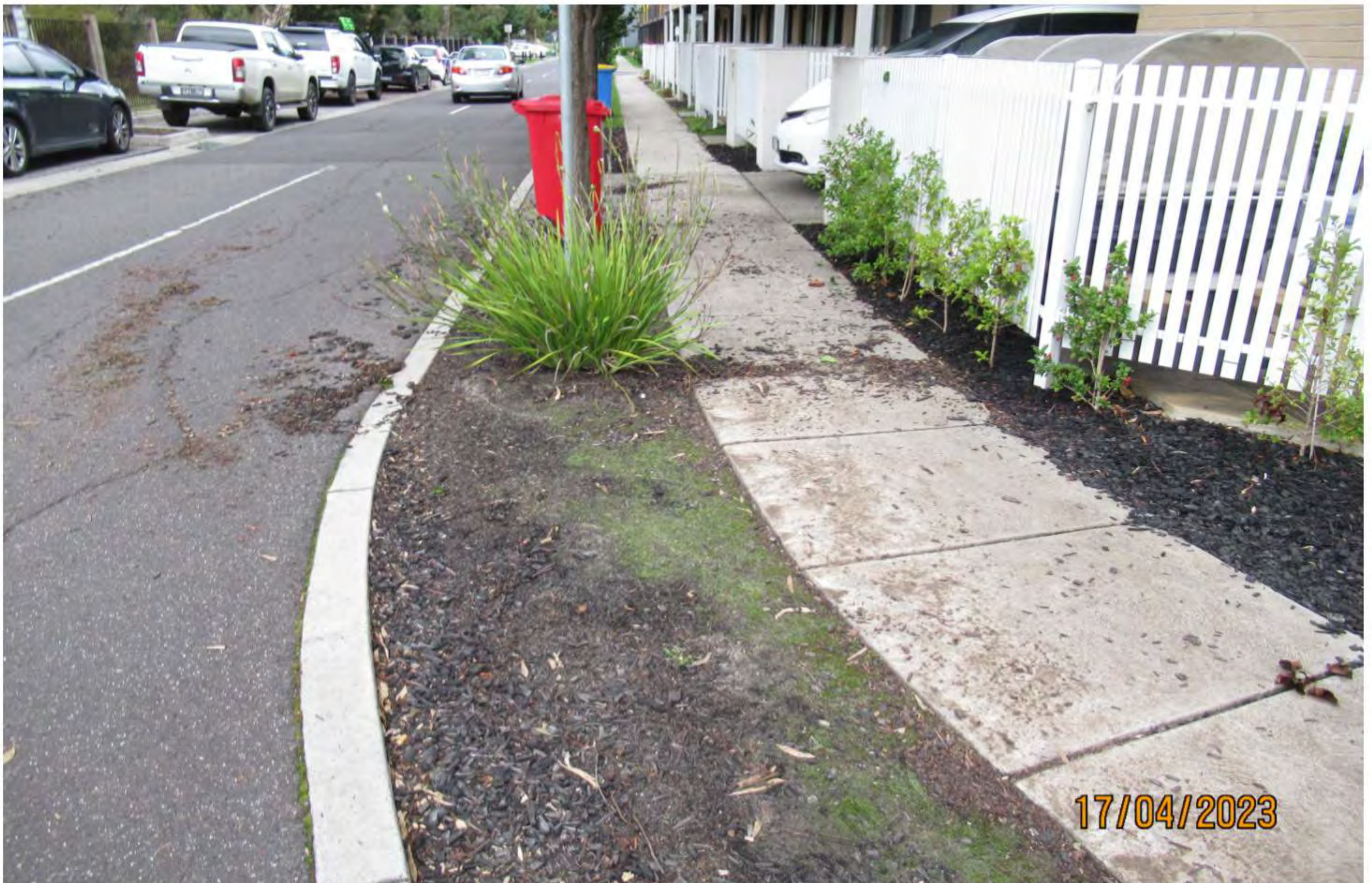
Photo 1.23: Visible signs of water inundation from leak
