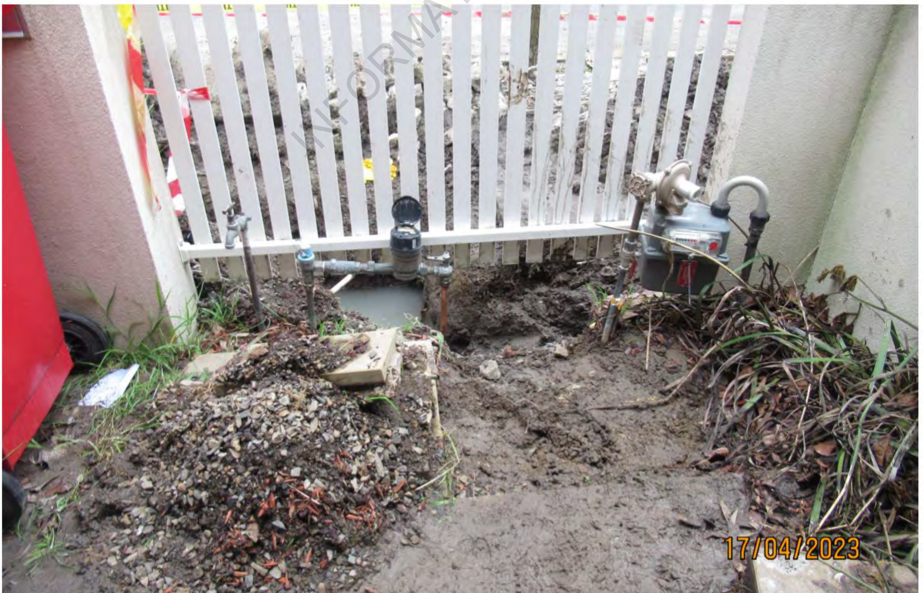
Photo 1.28: Repairs carried out to leaking water pipe
