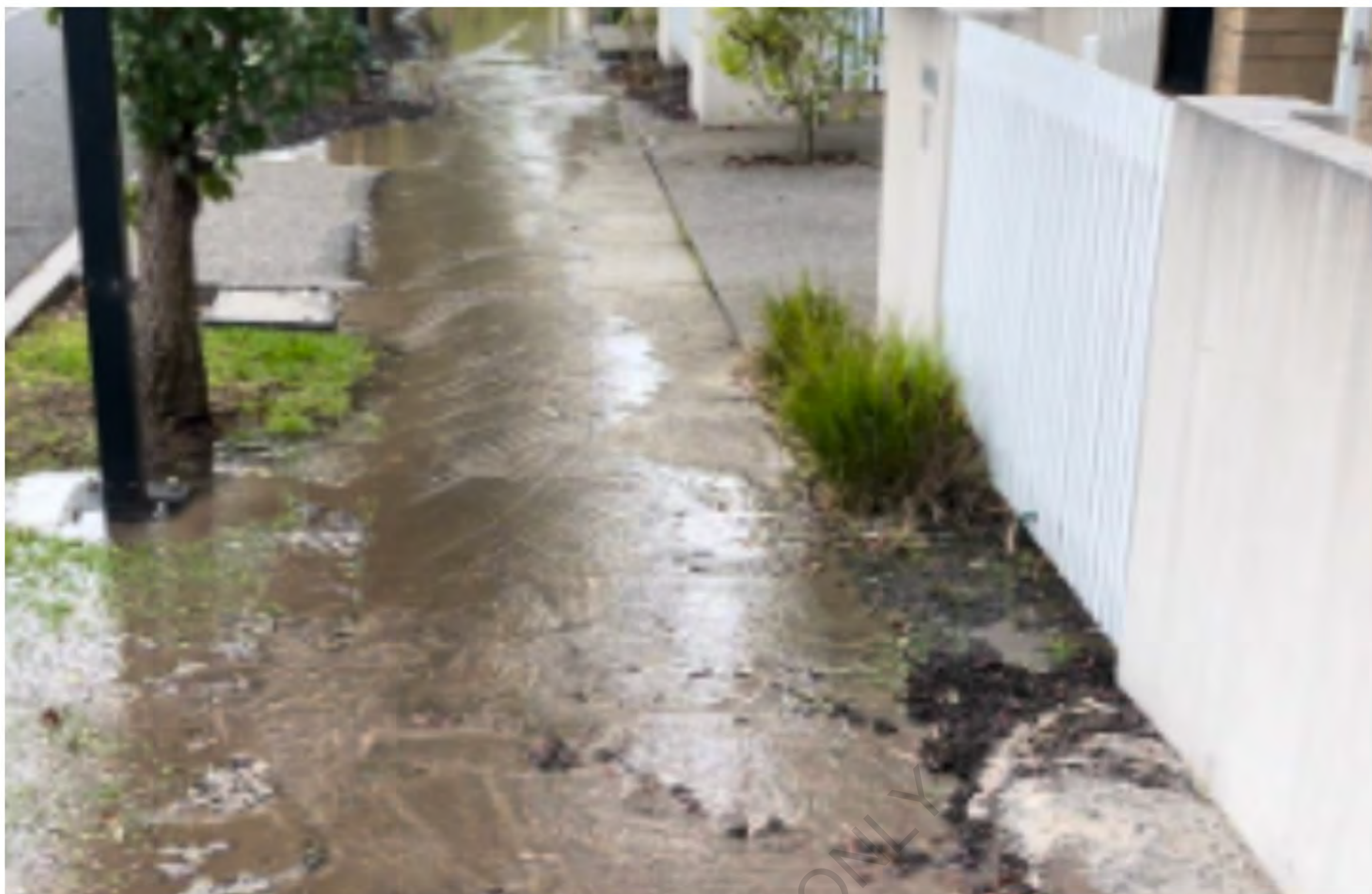
Photo 2.1: Water leakage from front of 10 Gorman Drive
