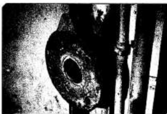
Figure 7: Asbestos-containing gasket.
