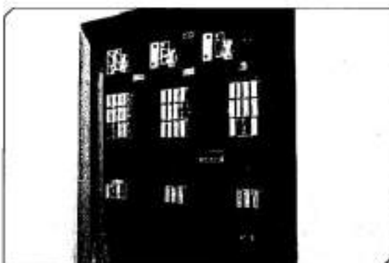
Figure 16: Asbestos-containing zirconite electrical switchboard panel.
