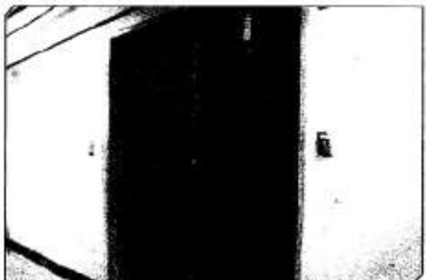
Figure 13: Fire-rated door containing asbestos.
