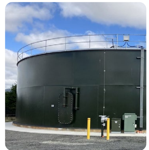
Upgrades to the Romsey Water Filtration Plant have started.
