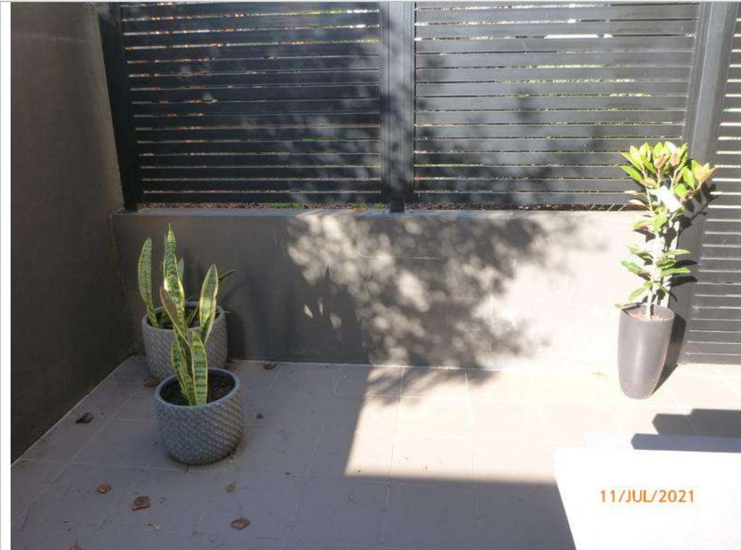
Photograph 27 – Terrace dividing wall
