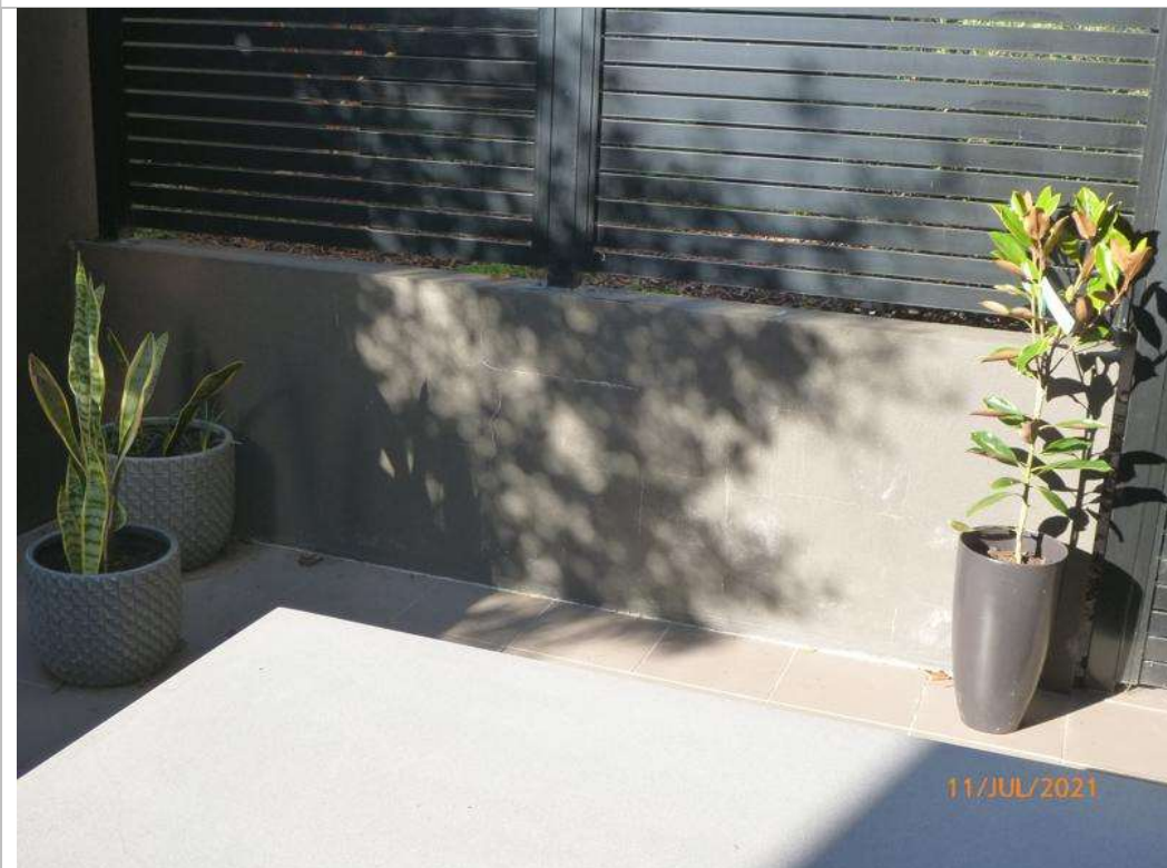
Photograph 28 – Terrace dividing wall
