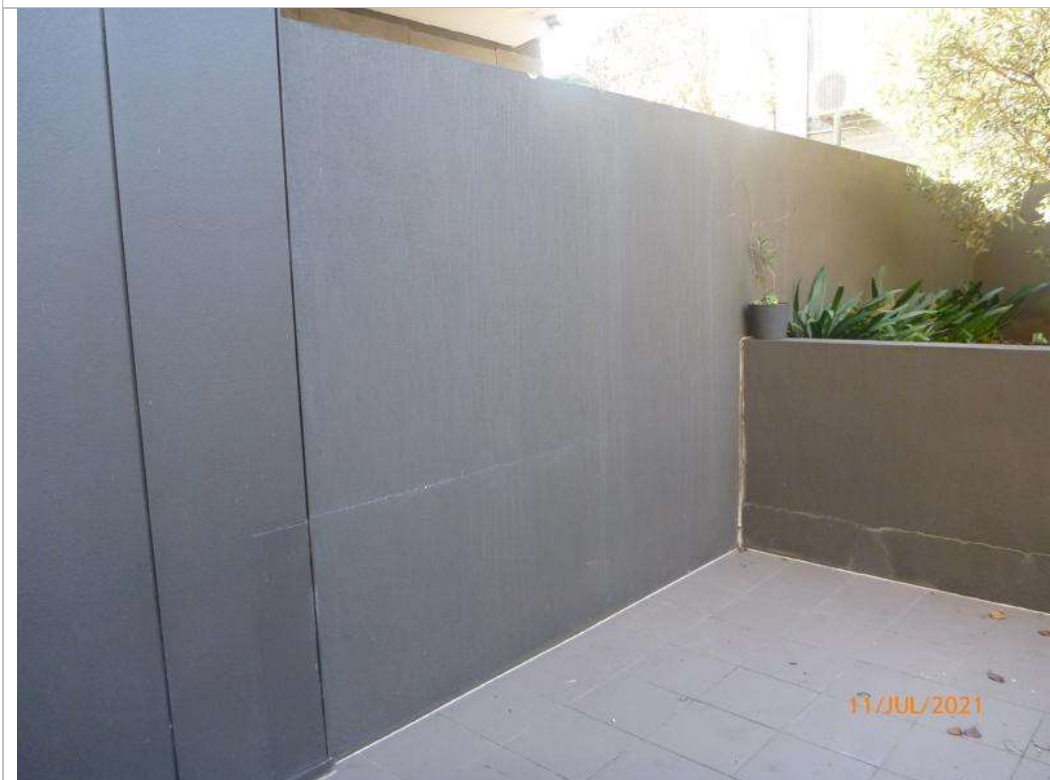
Photograph 26 – Terrace retaining walls
