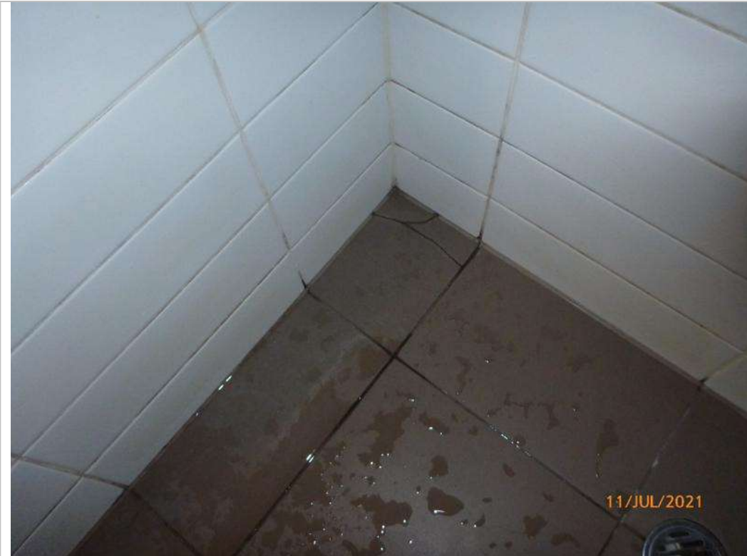
Photograph 3 – Bathroom shower base
