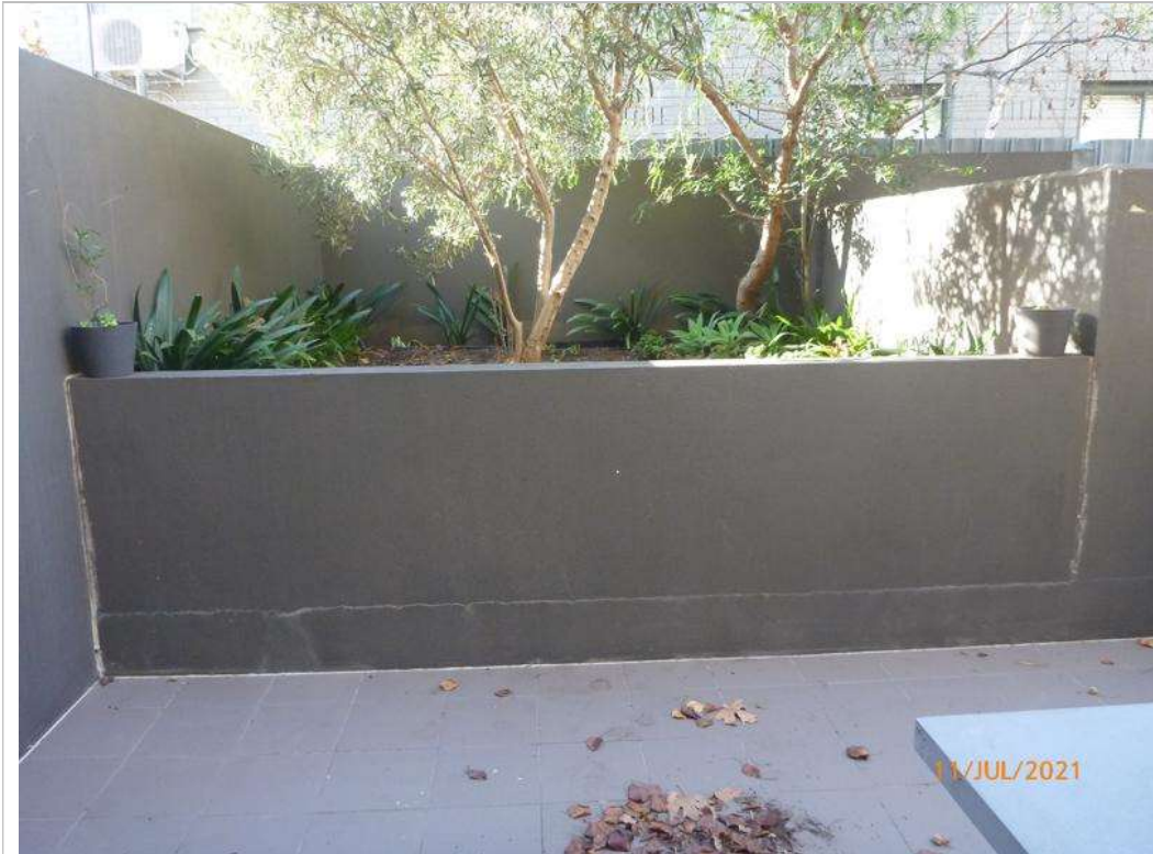
Photograph 25 – Terrace retaining walls
