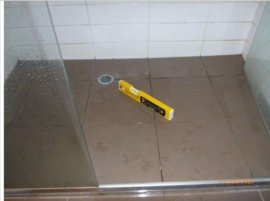
Photograph 5 – Bathroom shower base
