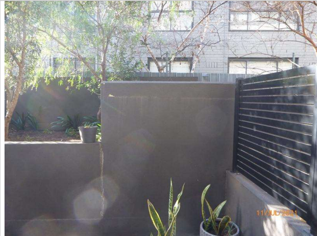
Photograph 23 – Terrace retaining walls
