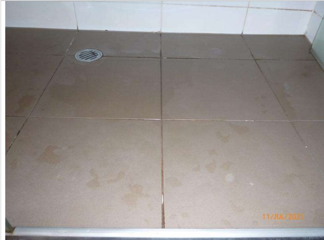
Photograph 7 – Bathroom shower base
