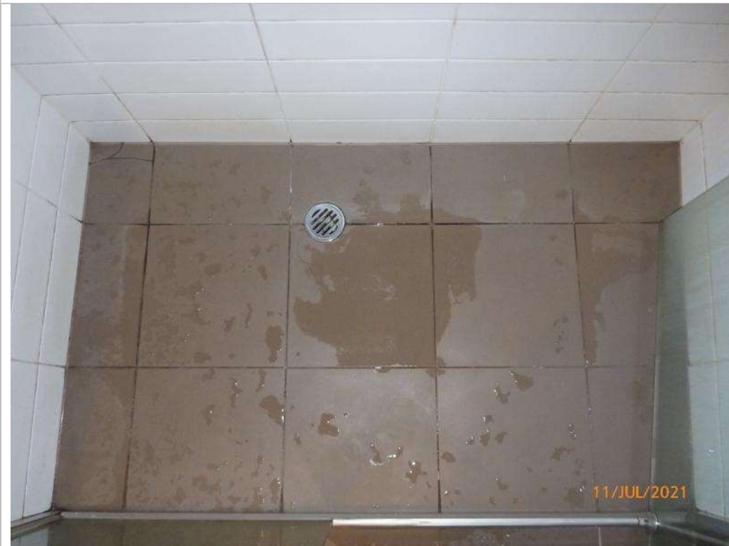
Photograph 2 – Bathroom shower base
