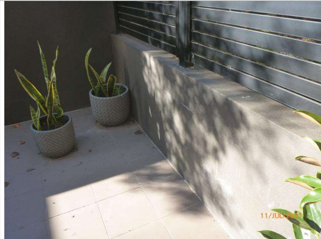
Photograph 29 – Rusted render corner beads
