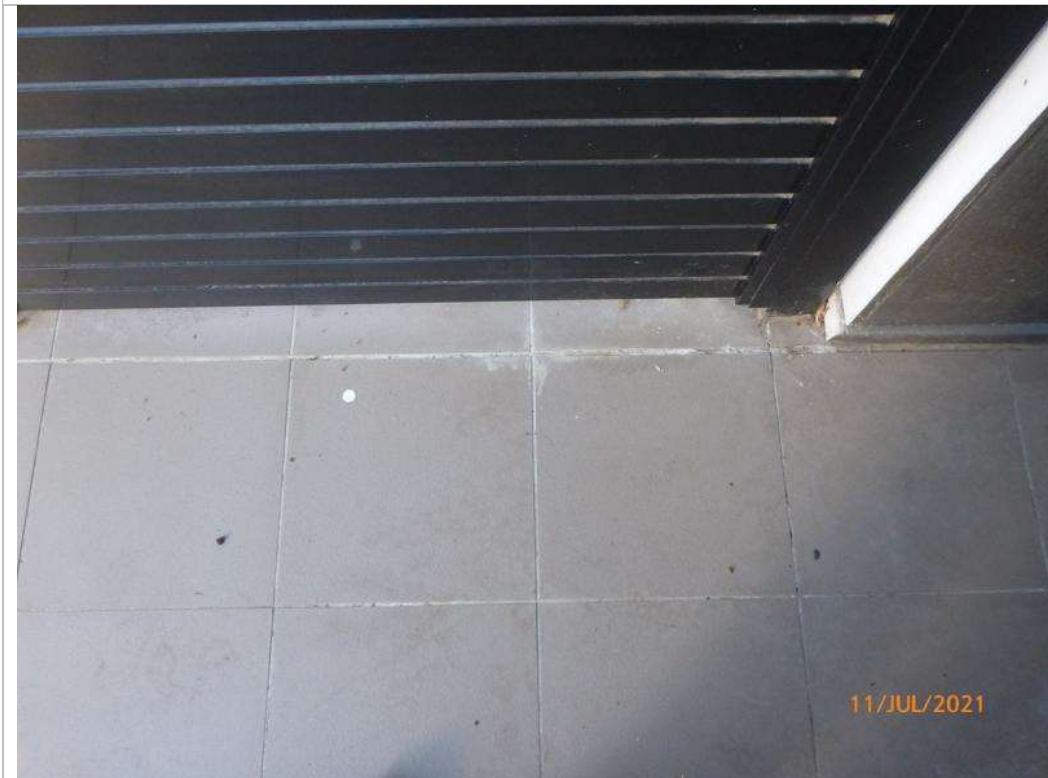
Photograph 18 – Terrace efflorescence
