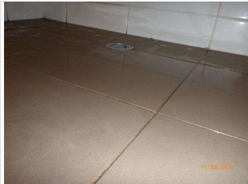
Photograph 8 – Bathroom shower base
