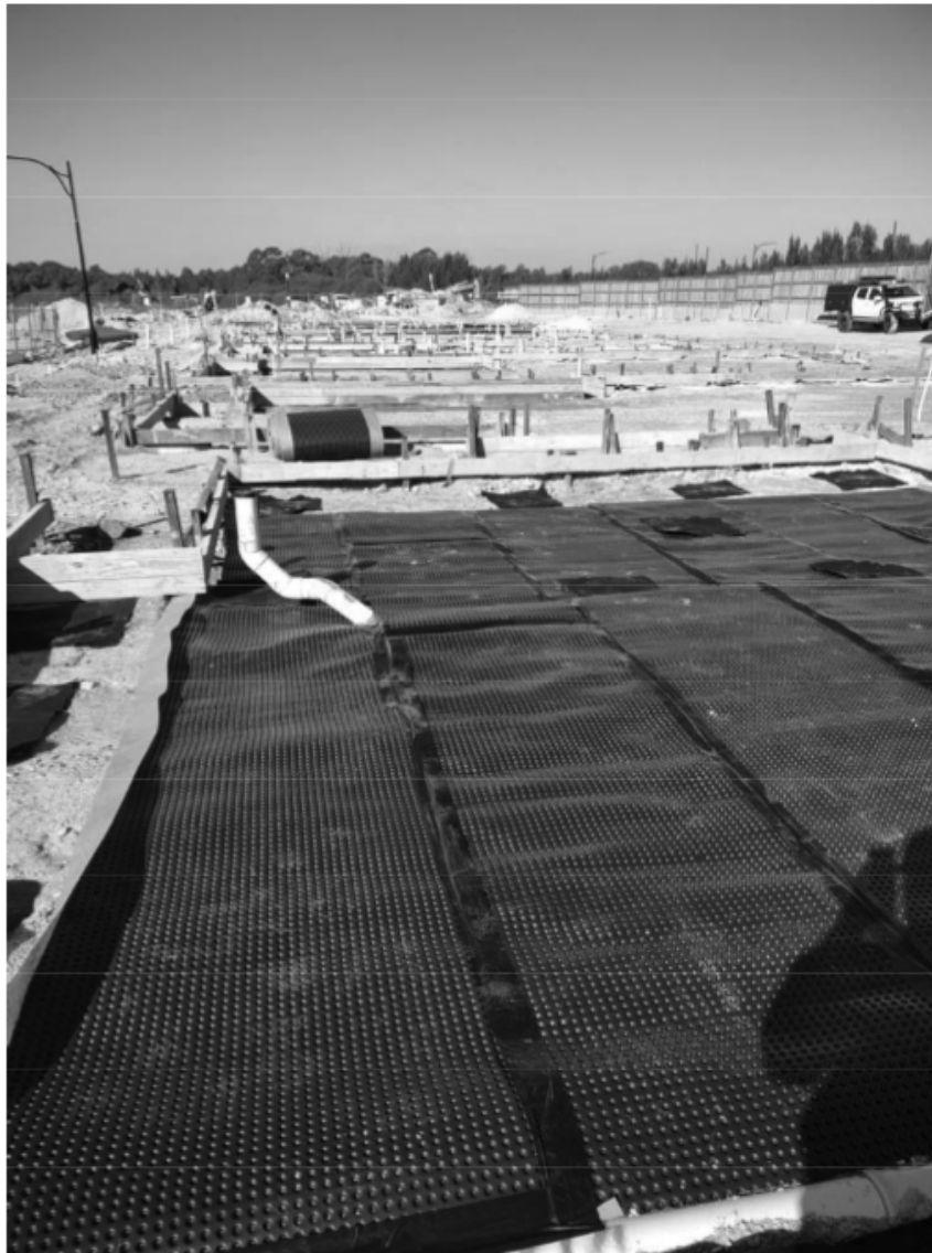
Figure 2: Gas drainage layer
