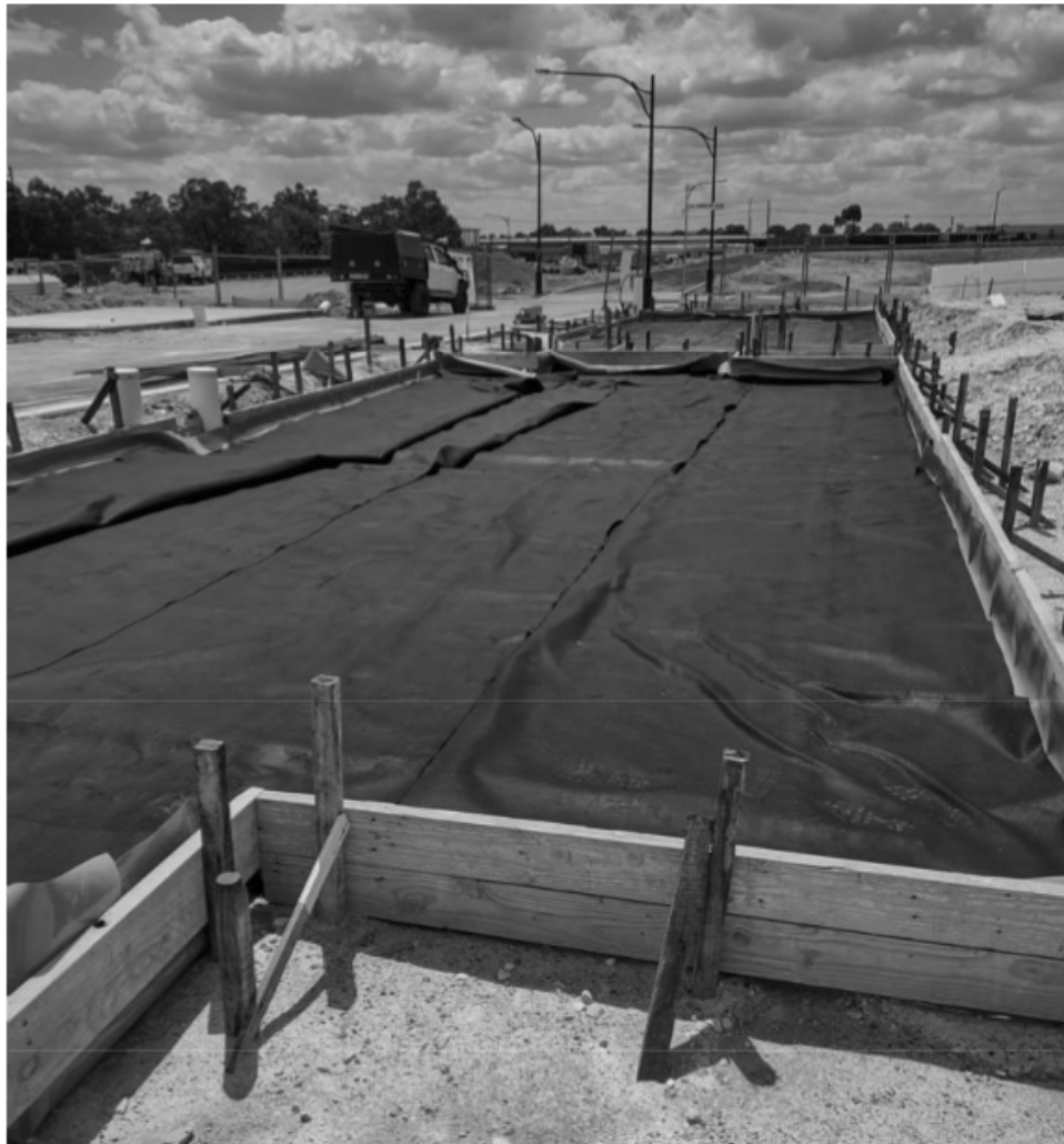
Figure 4: Geotextile protection layer
