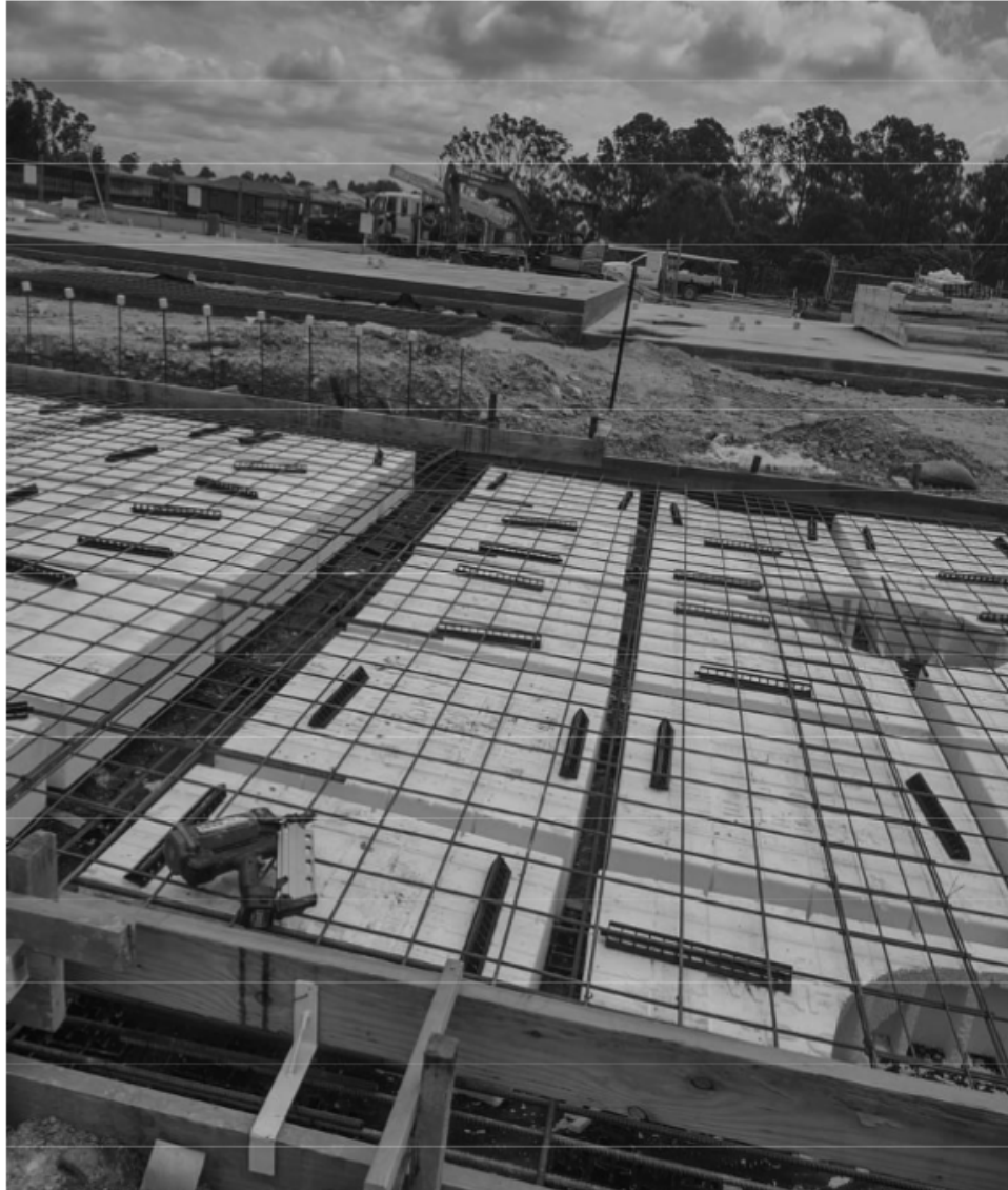
Figure 5: Concrete slab (steel reinforcement and waffle-pods placed over the geotextile, pre-concrete pour)
