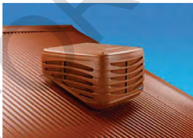
LOW PROFILE & POSITIONED AT REAR ACCEPTABLE
