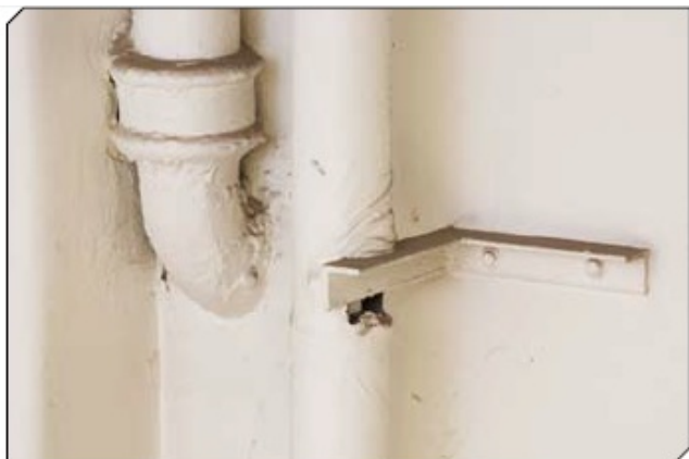
Figure 8: Damaged and exposed pipe wrapped with asbestos lagging.
