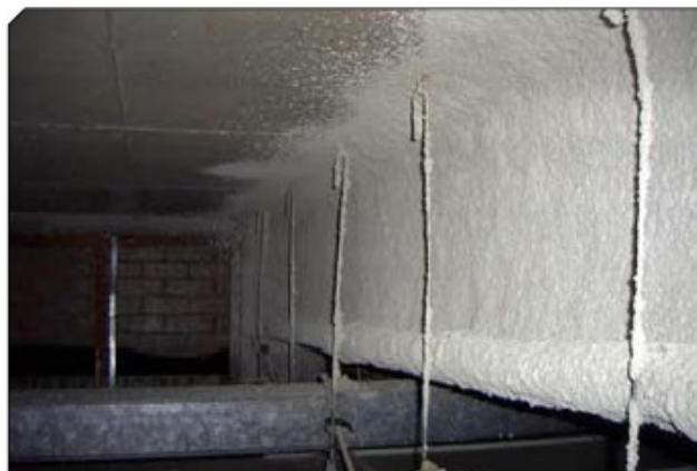
Figure 11: Sprayed asbestos.
