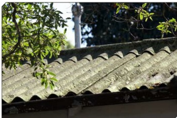
Figure 4: Corrugated asbestos cement roof sheets.
