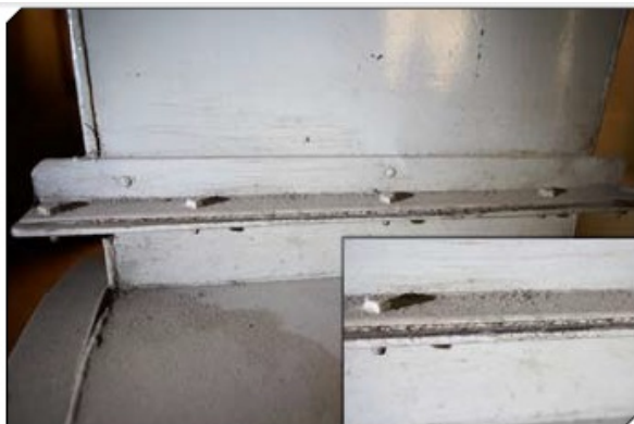
Figure 14: Asbestos rope seal in duct join with close-up inset
