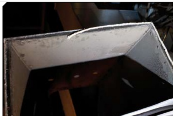
Figure 15: Detached asbestos rope seal and remnant debris on duct
