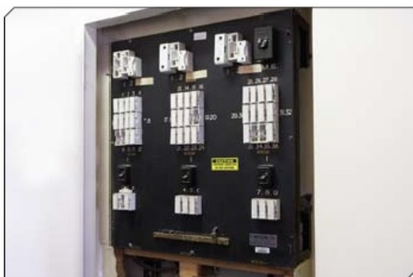
Figure 16: Asbestos-containing zelemite electrical switchboard panel.
