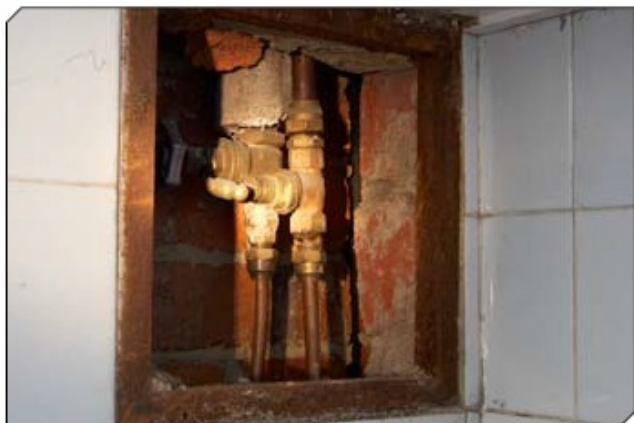
Figure 10: Exposed asbestos lagging on pipe.
