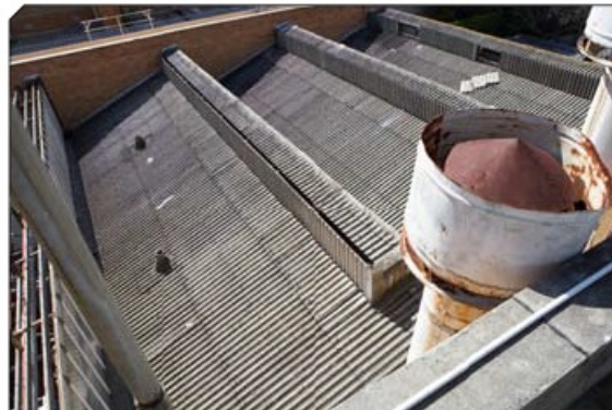
Figure 3: Corrugated asbestos cement roof sheets.
