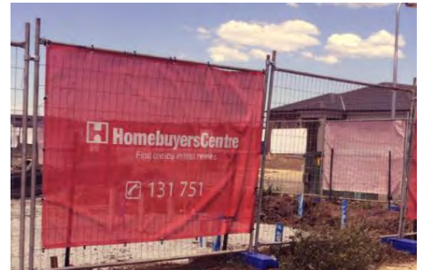
TEMPORARY CHAINLINK FENCE W/ - BANNER MESH
