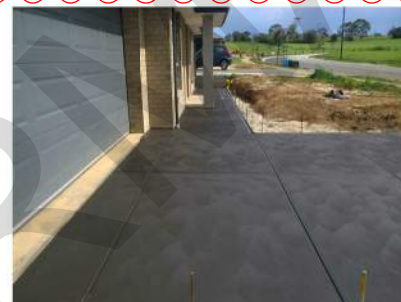
COLOUR THROUGH CHARCOAL COLOURED CONCRETE DRIVEWAY
