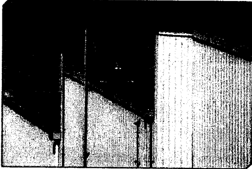
Figure 2: Saw-tooth design roof with corrugated asbestos cement roof sheets.
