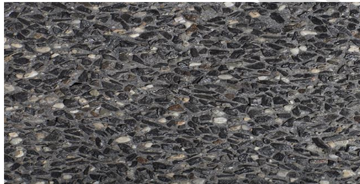
Example of exposed aggregate concrete.
