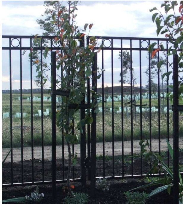
Figure 4.5 Typical Golf Lot Fencing Detail
